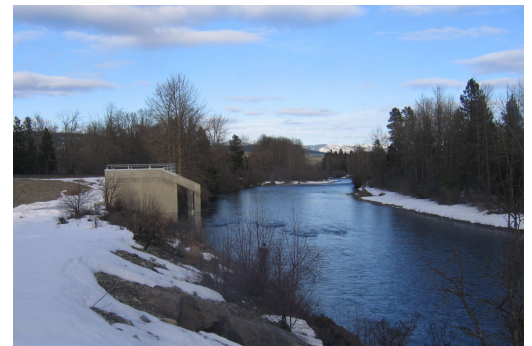
Example of a surface water intake structure
